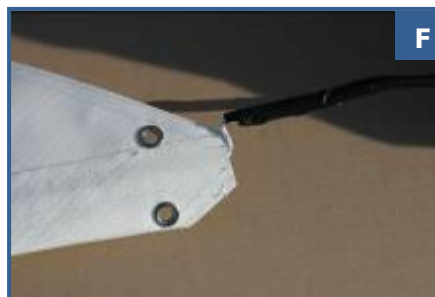
Scotcher le câble AT et le messenger ensemble / Tape together the AT rope and the messenger
