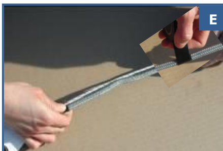
Scotcher le câble AT et le messenger ensemble / Tape together the AT rope and the messenger
